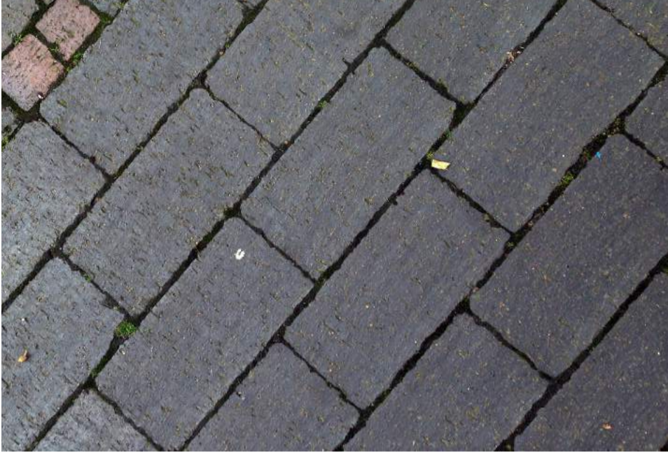
Clay sett paving
