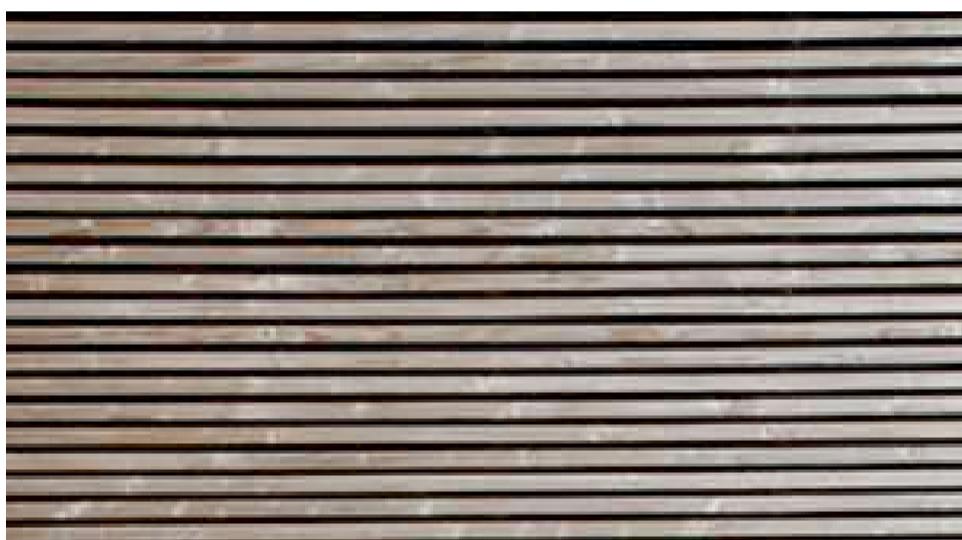
Untreated timber cladding
