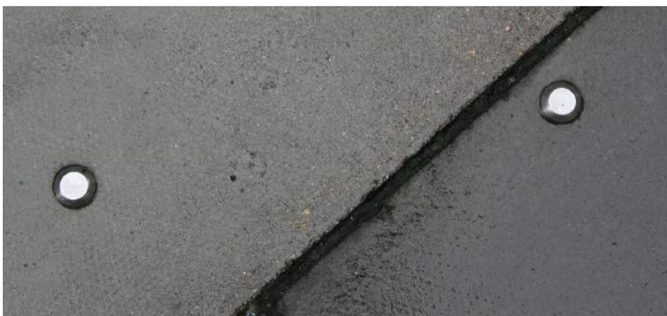
In-ground studs demarcating the stall layout
